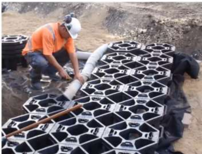
Strata cells store stormwater and make it available to trees in downtown environments, as seen on John Hirsh Place
