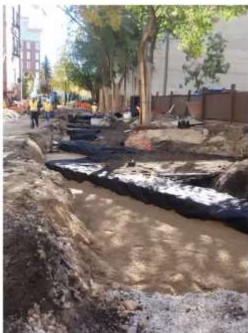
Strata cells store stormwater and make it available to trees in downtown environments, as seen on John Hirsh Place
