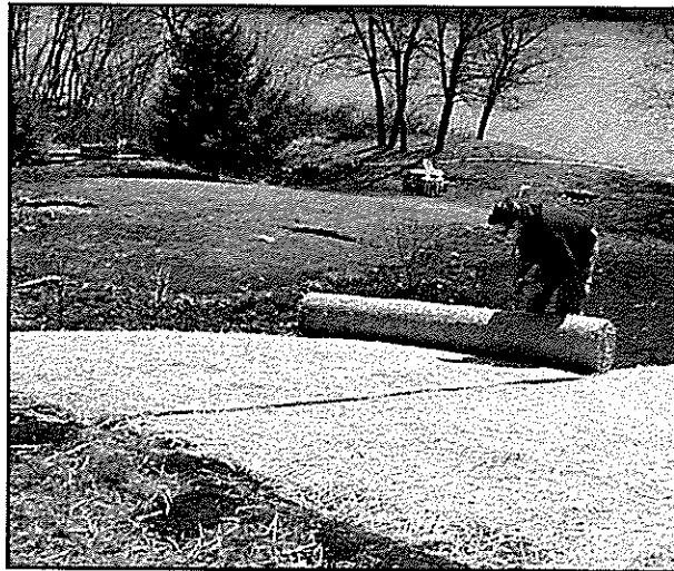
Artificial thatch over a seeded slope keeps the seed and soil out of waterways. Photo by Mark Myrowich
